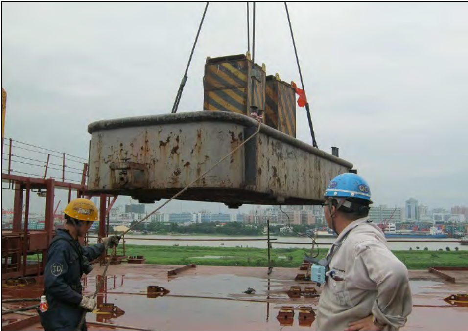
Weight used during Proof Testing
